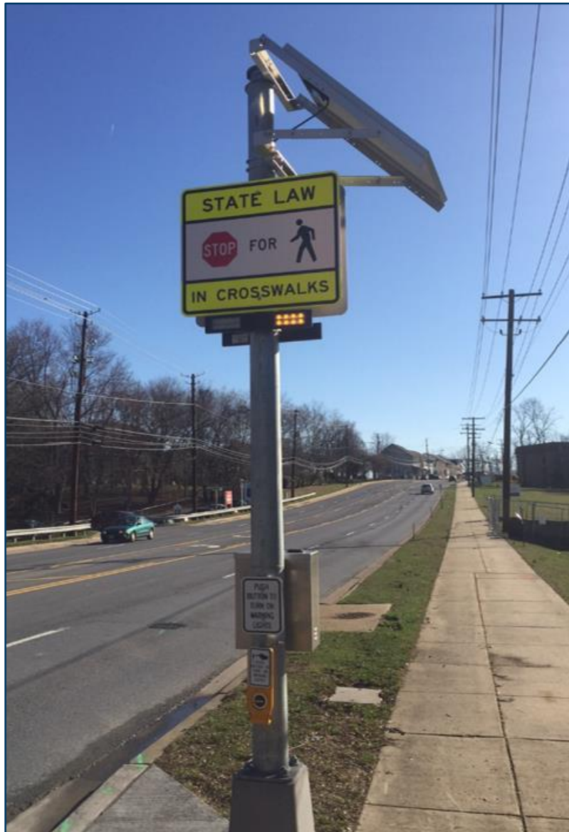
RRFB on Bel Pre Road
